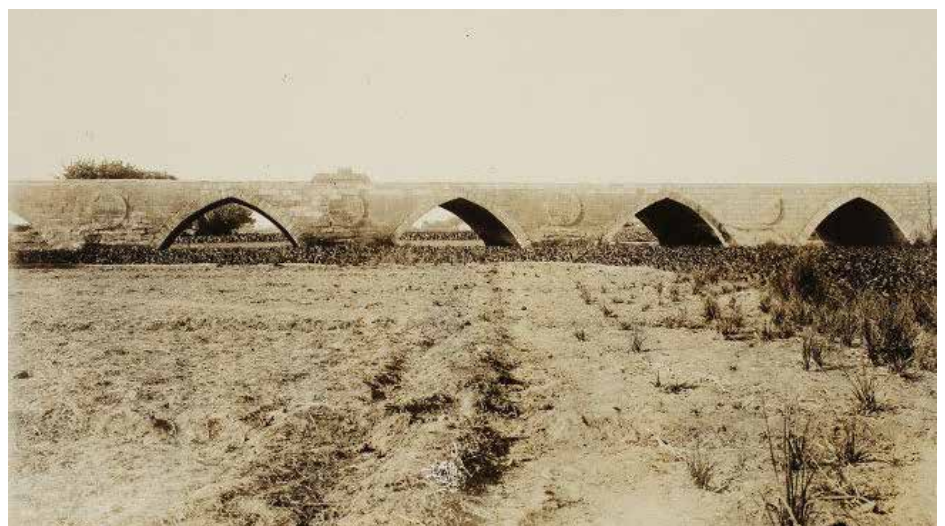
Figure 1: Bridge over the former Abū l-Munajja Canal which regulated the irrigation of the eastern Nile Delta, Cairo, 1260s. (Photo: K. A. C. Creswell, 1916-21, © Victoria and Albert Museum, London.)
